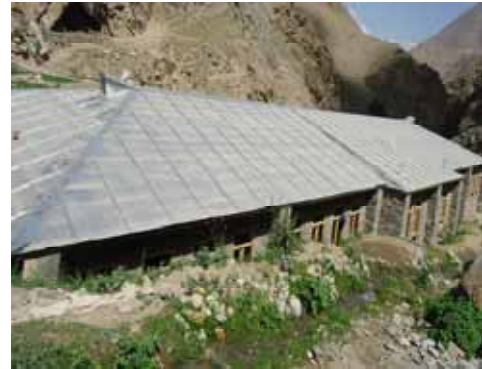
Yamgan School Constructed by EQUIP
