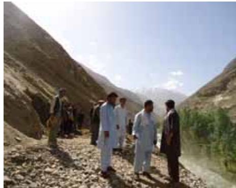
EQUIP team surveys road block on way to Yamgan
